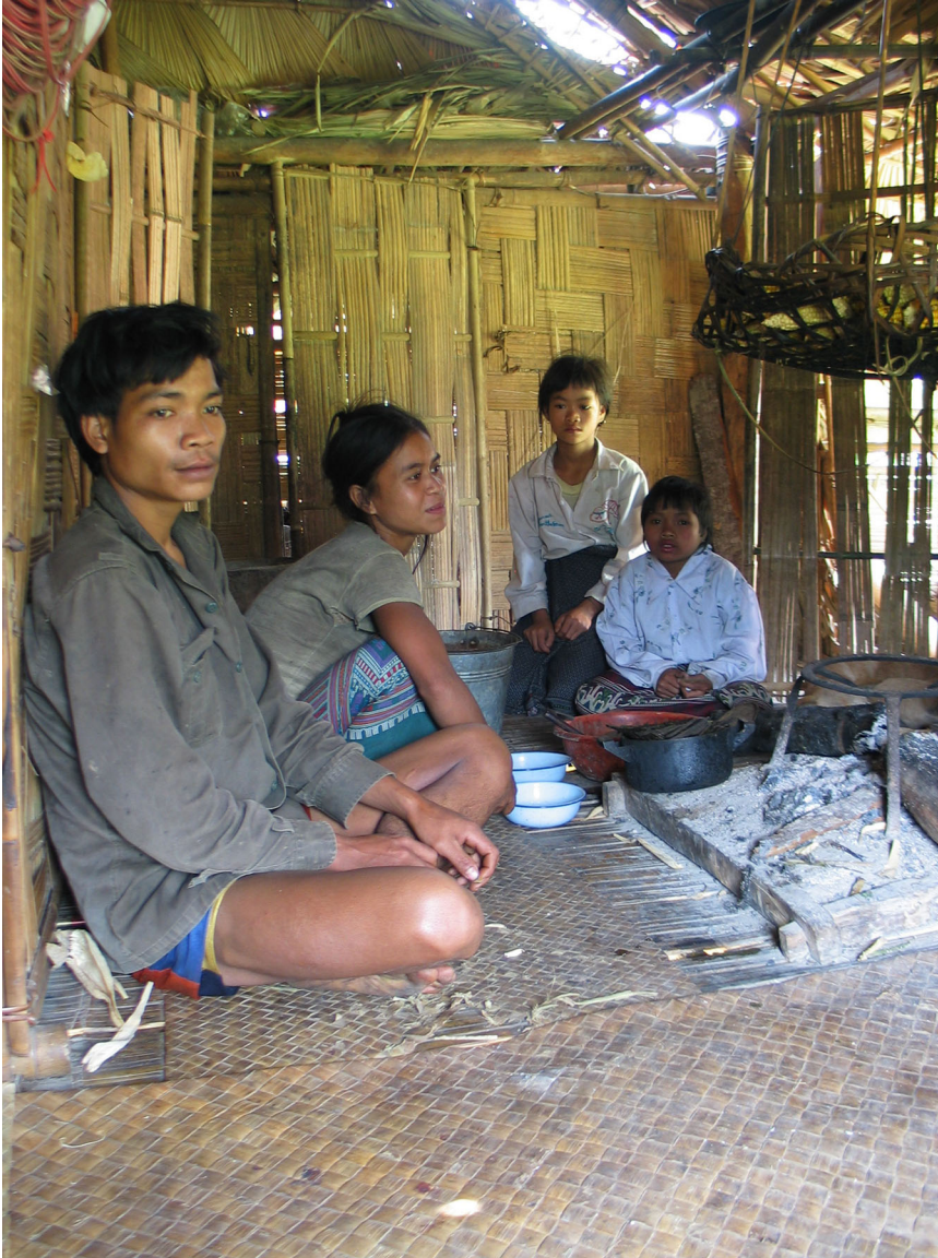
Figure 5. Interior with split-bamboo flooring, partly covered by pandanus mats; note cooking hearth in central living space, not in a separate kitchen area (Upstream Mrkaa, 2004). (Photograph by Nick Enfield.)
