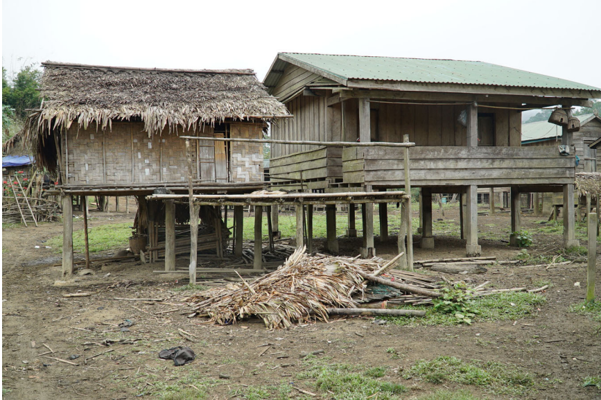
Figure 6. Timber house (Middle Mrkaa, 2018): at right, timber planks are used for wall panelling and floorboards; at left, a separate kitchen is constructed using materials normally used in a single-space Kri house (see Figs 3–5). (Photograph by Charles Zuckerman.)
