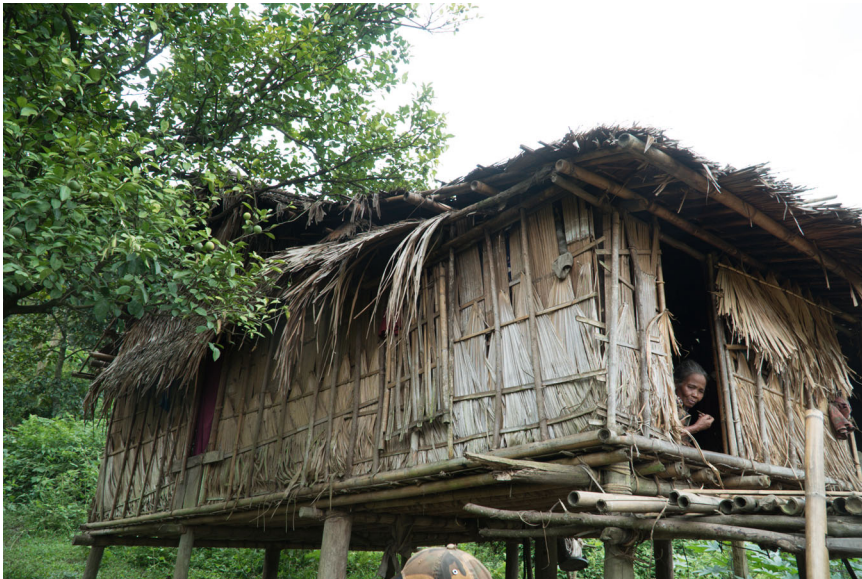
Figure 3. Exterior of a Kri traditional house in Upstream Mrkaa, 2018, made with machetes, using plant materials available in the forest neighbouring the village. (Photograph by Charles Zuckerman.)
